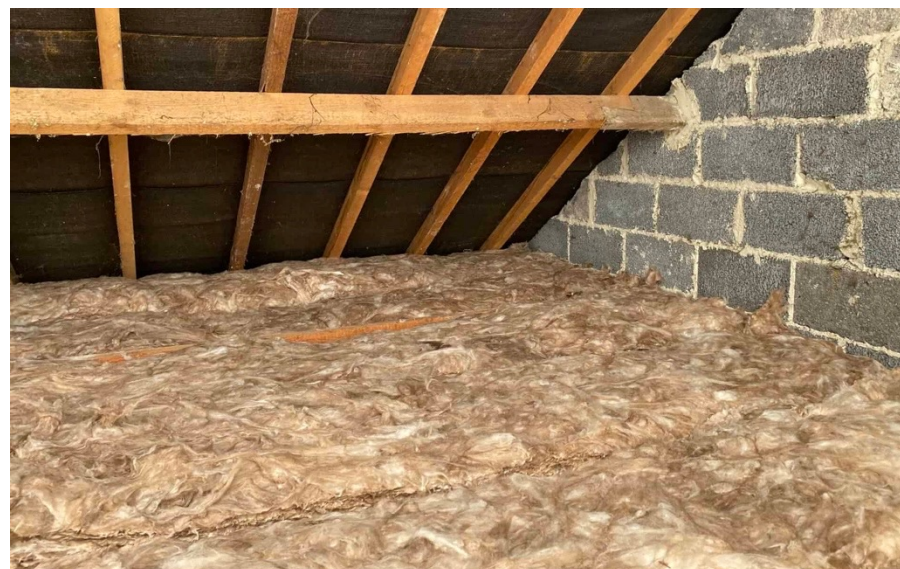
Ceiling level insulation is common in mass-built homes across the UK.
